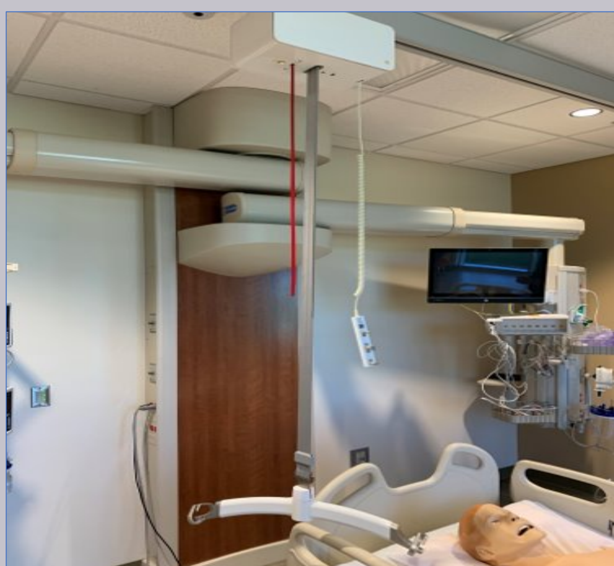
Figure 1: Ceiling lift system with hanger
